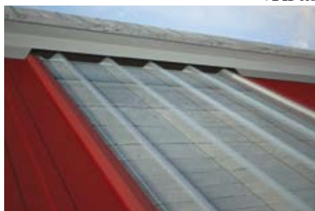
DETAIL OF RIDGE Detail of ridge with PE-LD seal
