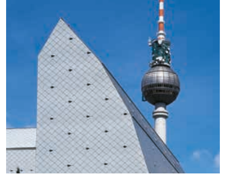
Berlinwasser Holding AG Binası, Berlin, Almanya
